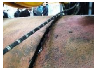
Cutting with diamond wire saw
