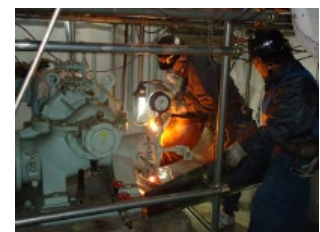
Verification of dismantling actual equipment and materials
