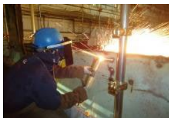
Cutting using gasoline
